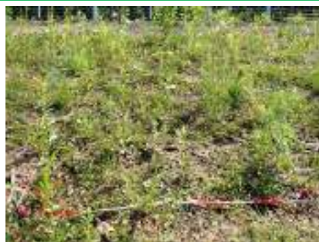
盛土法面の状況 (R5,植被率40%)
